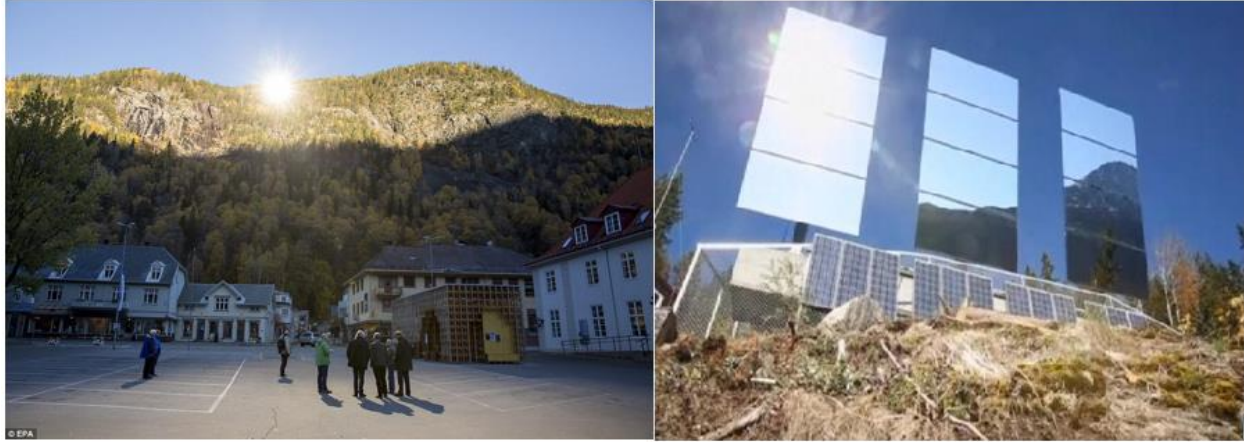
Fig. 3.4.2: An example of a heliostat in Rjukan, Norway. 7 Left: Mirrors reflect light from mountaintop. Right: Close view of the heliostat station. 8
